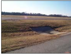
Know where the drains lead.
